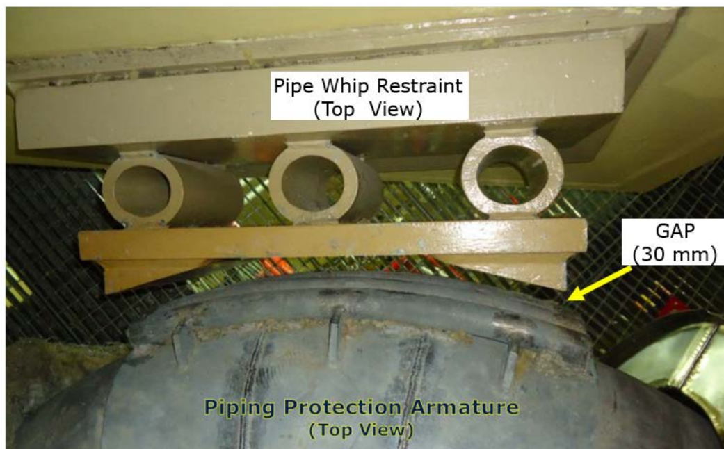
Figure 19: Top view of PWR in cold mode
