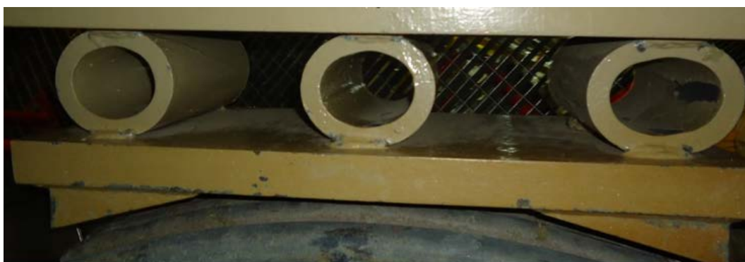
Figure 17: deformed pipe whip Restraints (top view)
