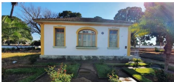
(a) Fachada principal
