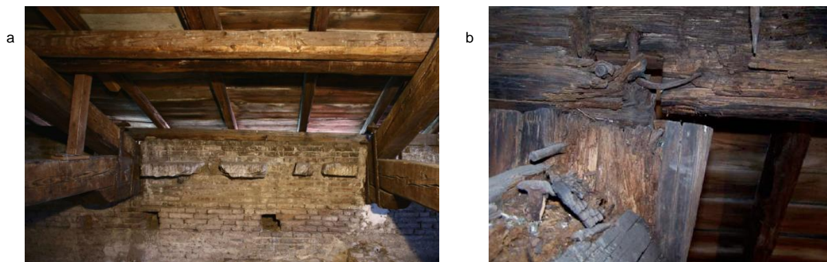
Figure 7. (a) Truss end supports; (b) Post-rafters connection
