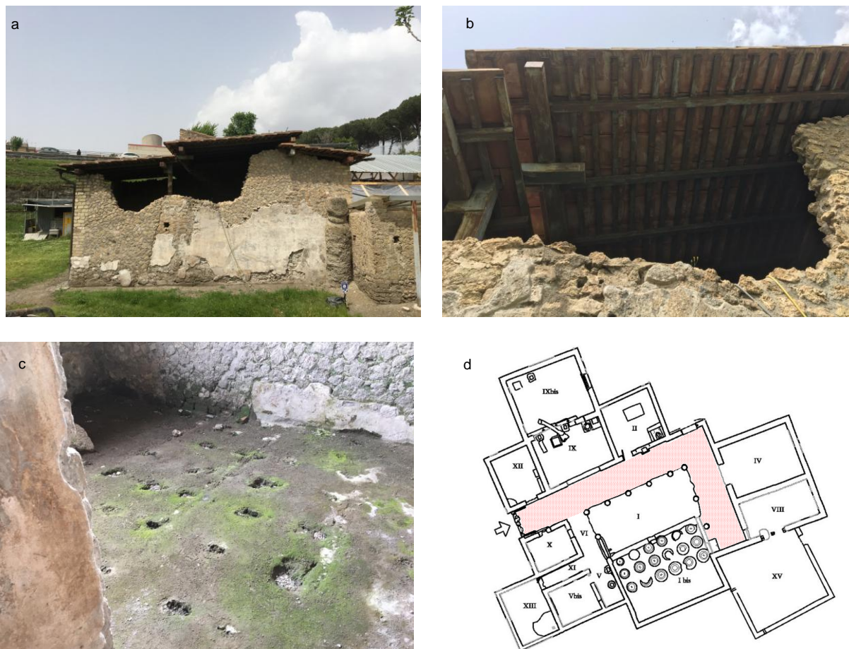
Figure 11. (a) North view of Villa Regina; (b) Detail of the roof; (c) Effects of leaching by rainwater; (d) plan of the villa
