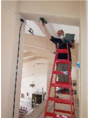
Figura 8: Reinforcement detection
