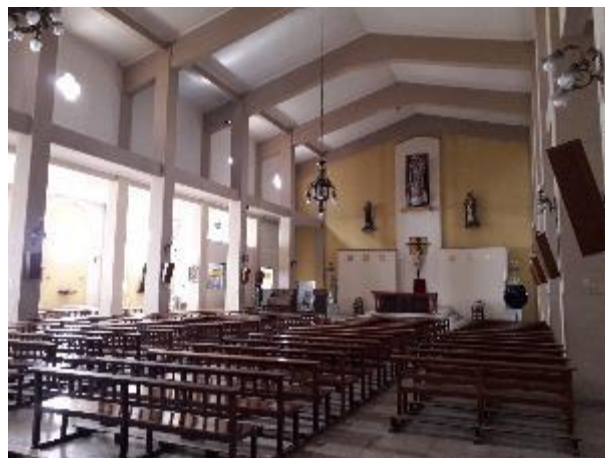
Figure 2: Interior view of the building in study
