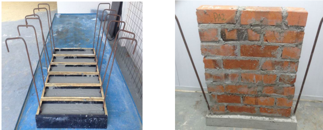
Figure 2. (a) Wall base and (b) Finished wall.
