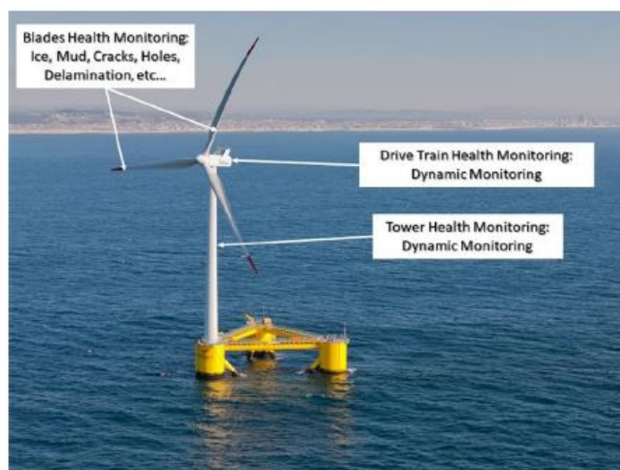
Figure 21: wind power monitoring system linked to DS [38]
