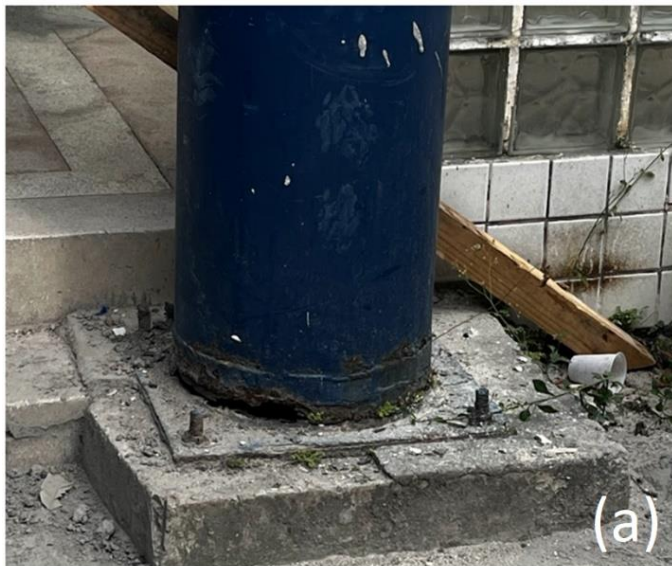
Figure 8 – Corrosion of the base of metal pillar (a) and corrosion of the distribution panel (b)
