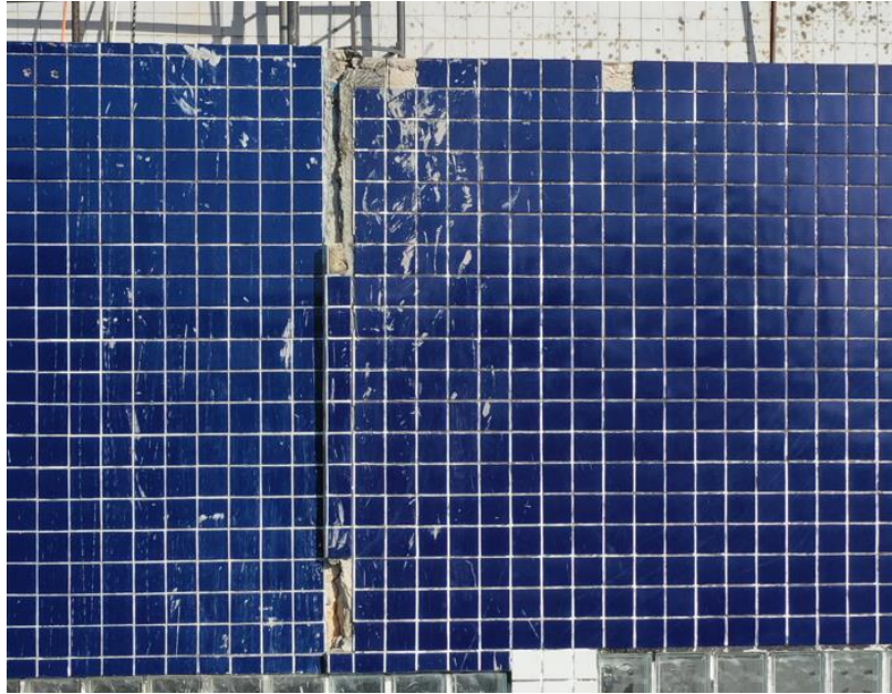
Figure 5 – Grime stains and ceramic detachment
