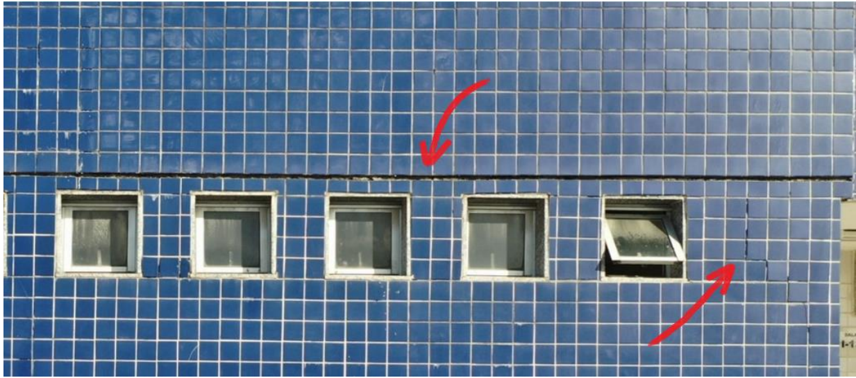
Figure 7 – Grout separation
