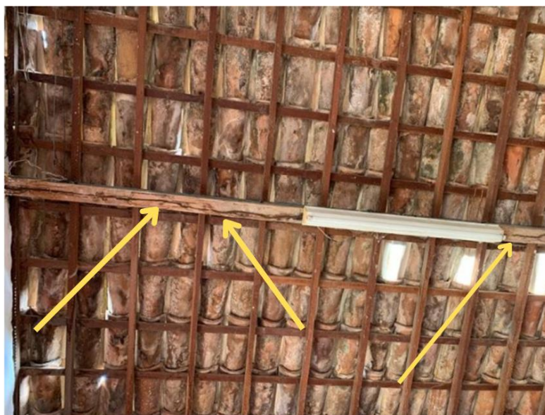
Figure 4 - Roof of the Hall of the Sacred Heart of Jesus
