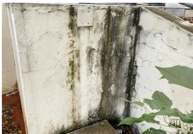
Figure 7 - Visual aspects of the presence of mold/biofilm caused by the absence of the marquee
