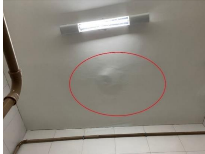
Figure 12 – Concrete expansion
