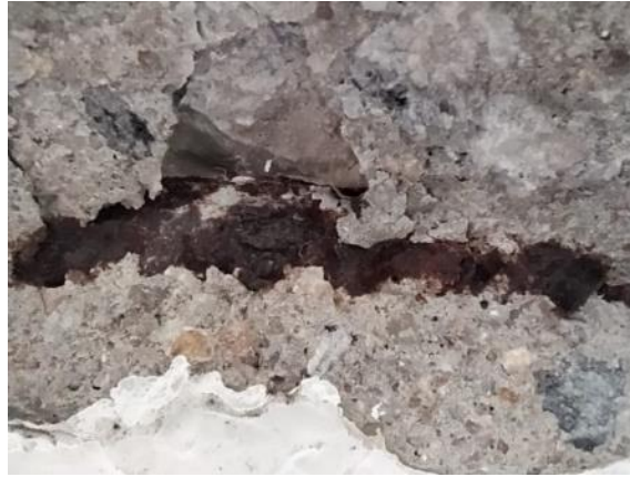
Figure 15 – Exposed rebar
