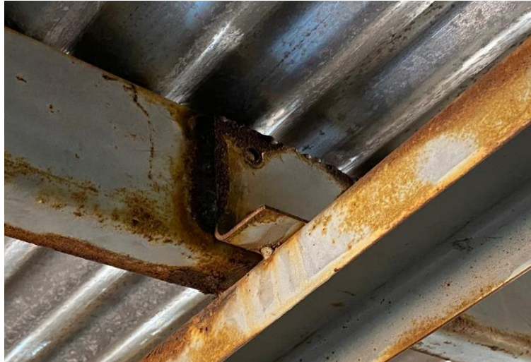
Figure 7 – Crevice corrosion
