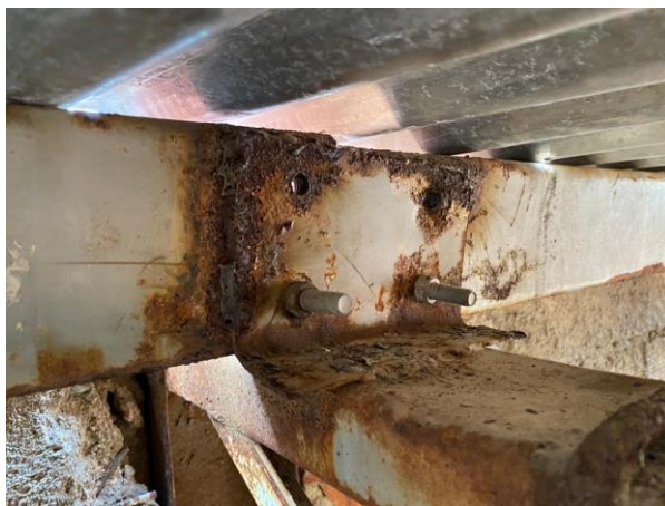
Figure 6 – Crevice corrosion
