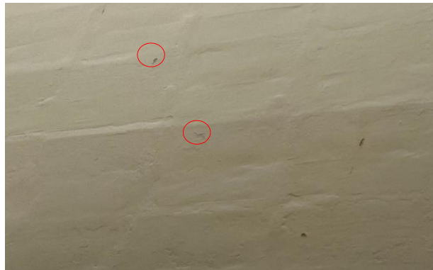
Figure 20 – Paint detachments
