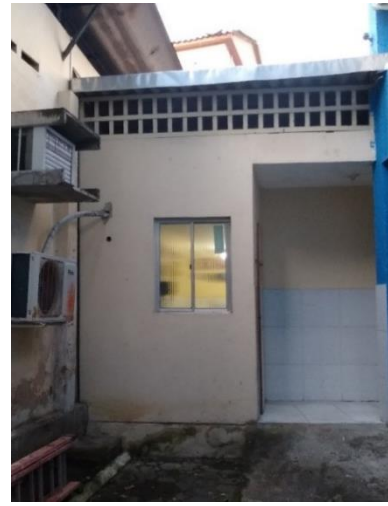
Figure 4 – Entrance to the laboratory
