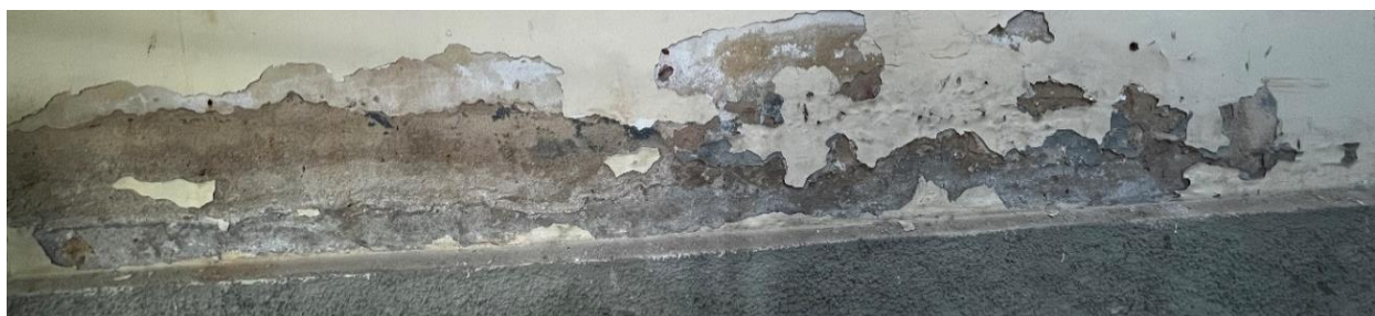
Figure 7 – Paint detachments
