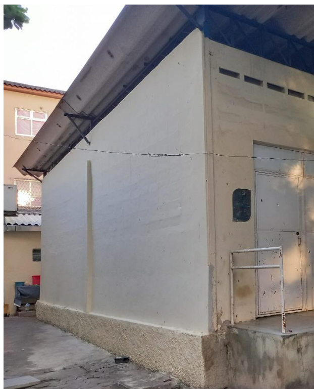
Figure 19 – Left side façade
