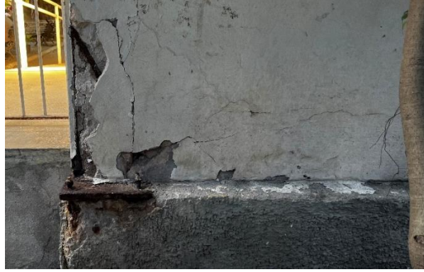
Figure 15 – Pillar of the right side façade
