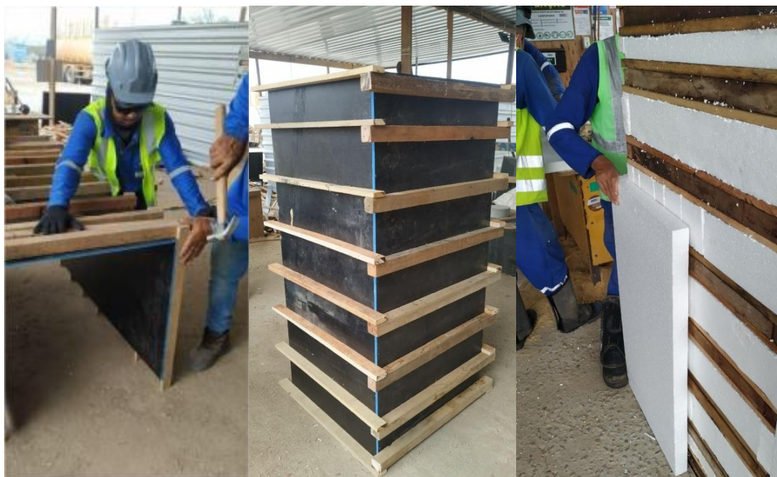
Figure 1 – Preliminary steps for performing thermal insulation with expanded polystyrene sheets, layers of plasticized wood and sealing with acetic silicone adhesive
