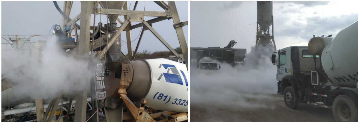
Figure 3 – Application of liquid nitrogen for the cooling of concrete aggregates
