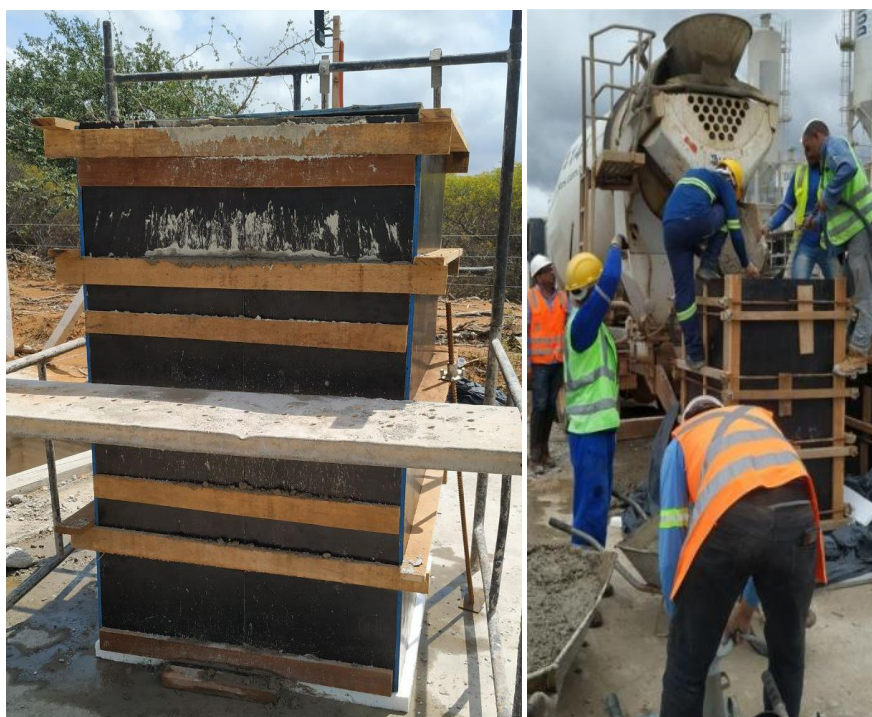
Figure 2 – Final disposition of the block isolated with EPS and execution of block concreting with mechanical vibration
