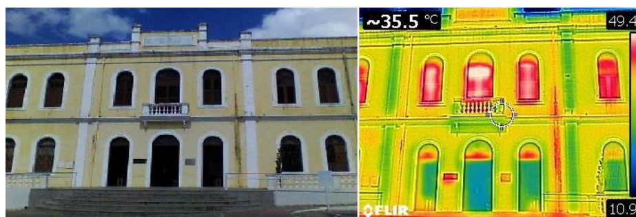
Figure 19 - Thermographic map of the Vale do Acaraú State University (UVA) - Betânia Campus facade in the morning.
