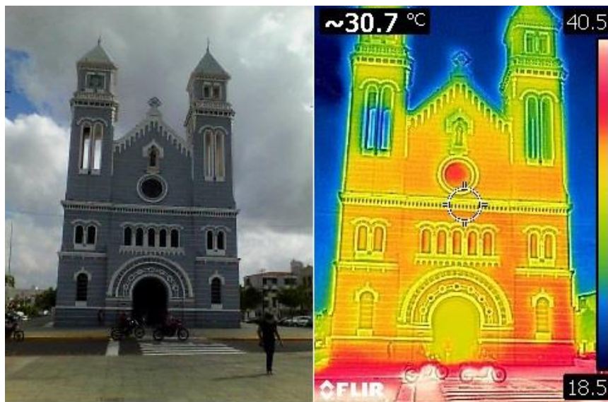
Figure 9 - Thermographic map of the facade of São Francisco Church in the morning.
