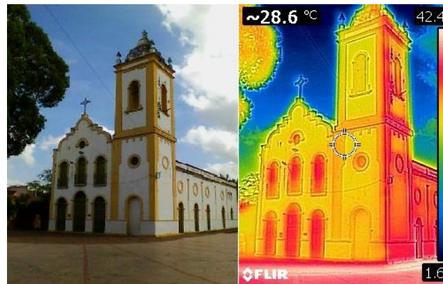
Figure 6 - Thermographic map of the facade of Church of Sorrows in the morning.
