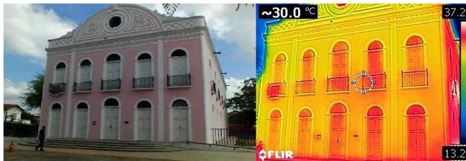
Figure 3 - Thermographic map of the facade of São João Theater in the morning.
