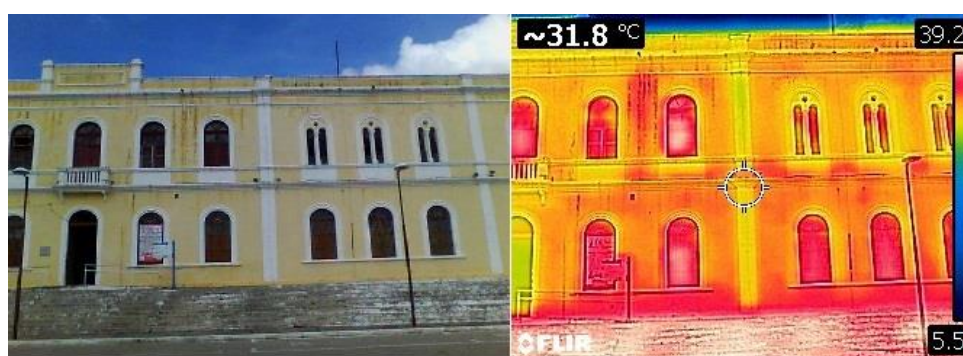
Figure 21 - Thermographic analysis of an outcrop on the facade of Campus Betânia- Vale do Acaraú State University (UVA).
