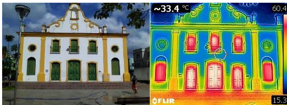
Figure 12 - Thermographic map of the facade of Church of the Rosary in the morning.
