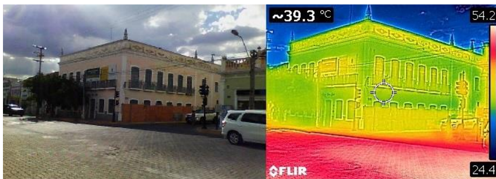
Figure 15 - Thermographic map of the facade of the Dom José Museum in the morning.
