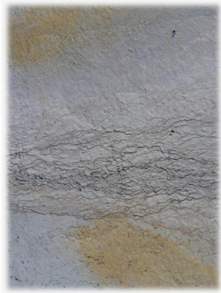
Figure 7 – Example of concrete segregation in a wind turbine foundation.
