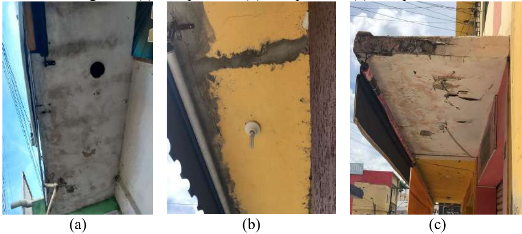
Figura 5. (a) Marquise 01, (b) Marquise 02, (c) Marquise 03
